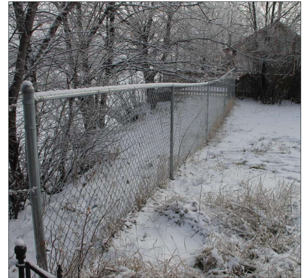
Rear Yard – 263 Houston Ave
